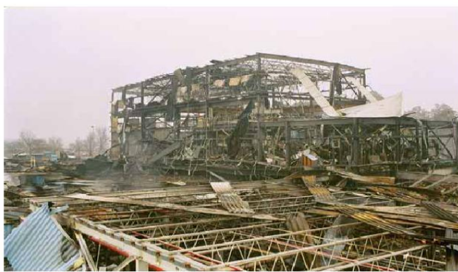
Figure 4. West Pharmaceutical Services facility destroyed by polyethylene dust explosion 13
